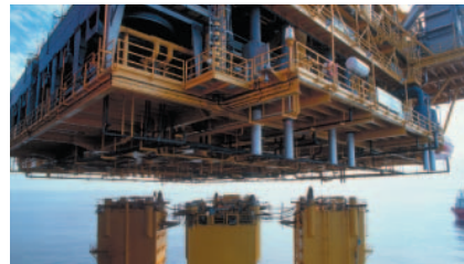
Offshore integration of deck and hull (Marco Polo TLP)
